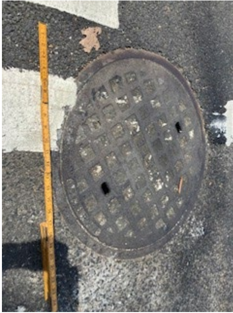
Photos below of utility hole in crosswalk
