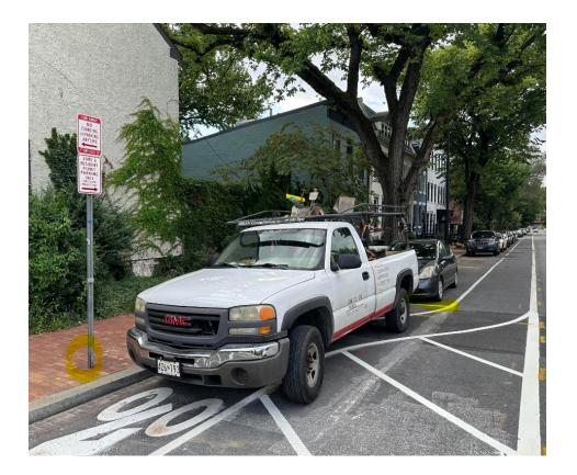
Photo of east side of 700 block 11<sup>th</sup> Street, SE before the G Street intersection. Bike lane markings have been altered, but No Parking signs have not been moved – so parked cars are blocking the revised bike lane markings, forcing cyclists to move into unprotected lanes. This incomplete modification has increased safety risks to cyclists and pedestrians at this intersection. Each NOIs identifies 4 revisions to the parking spaces and signs and none have been executed.
